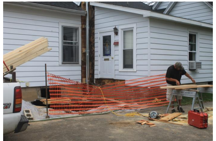
Replacing the Basement/Bilco Doors
